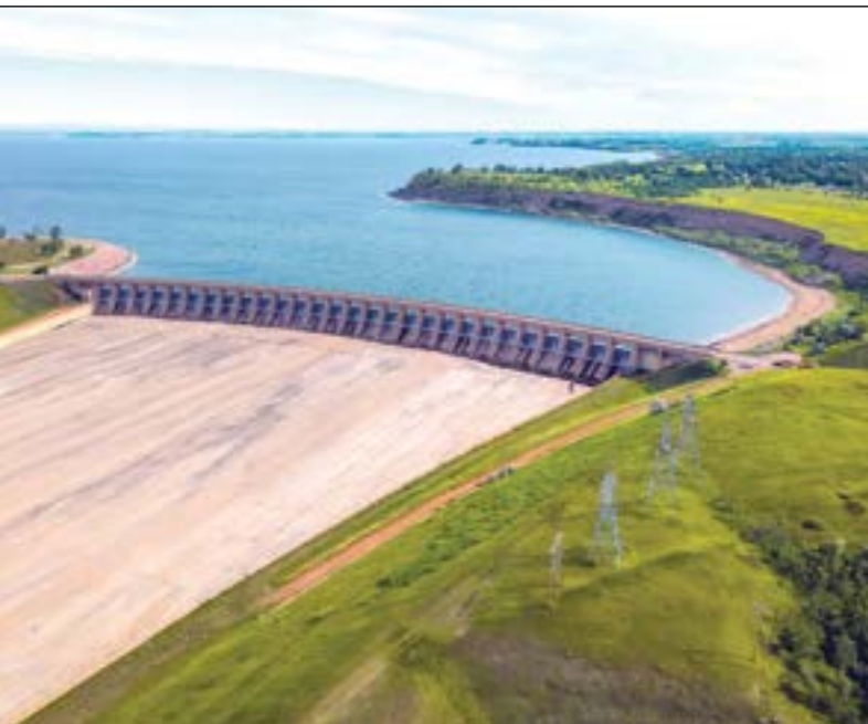
Garrison Dam at Lake Sakakawea in North Dakota.
