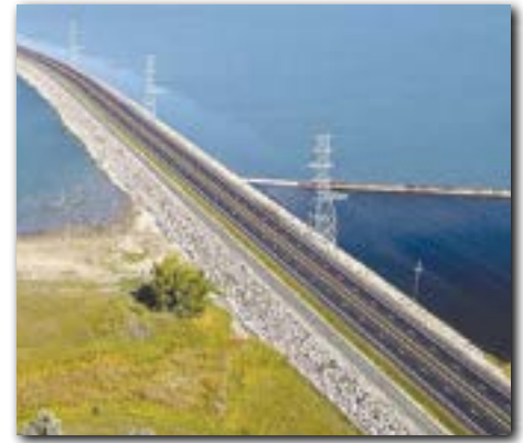
Snake Creek Embankment
