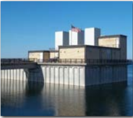
Snake Creek Pumping Plant
